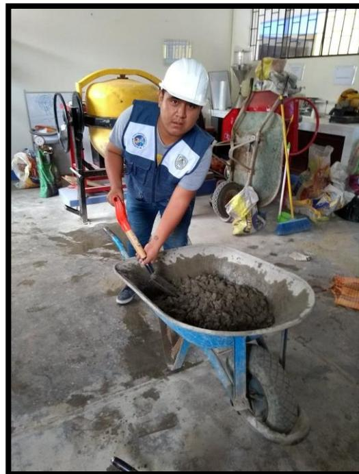
**FIGURA 26: MEZCLA DEL CONCRETO**
